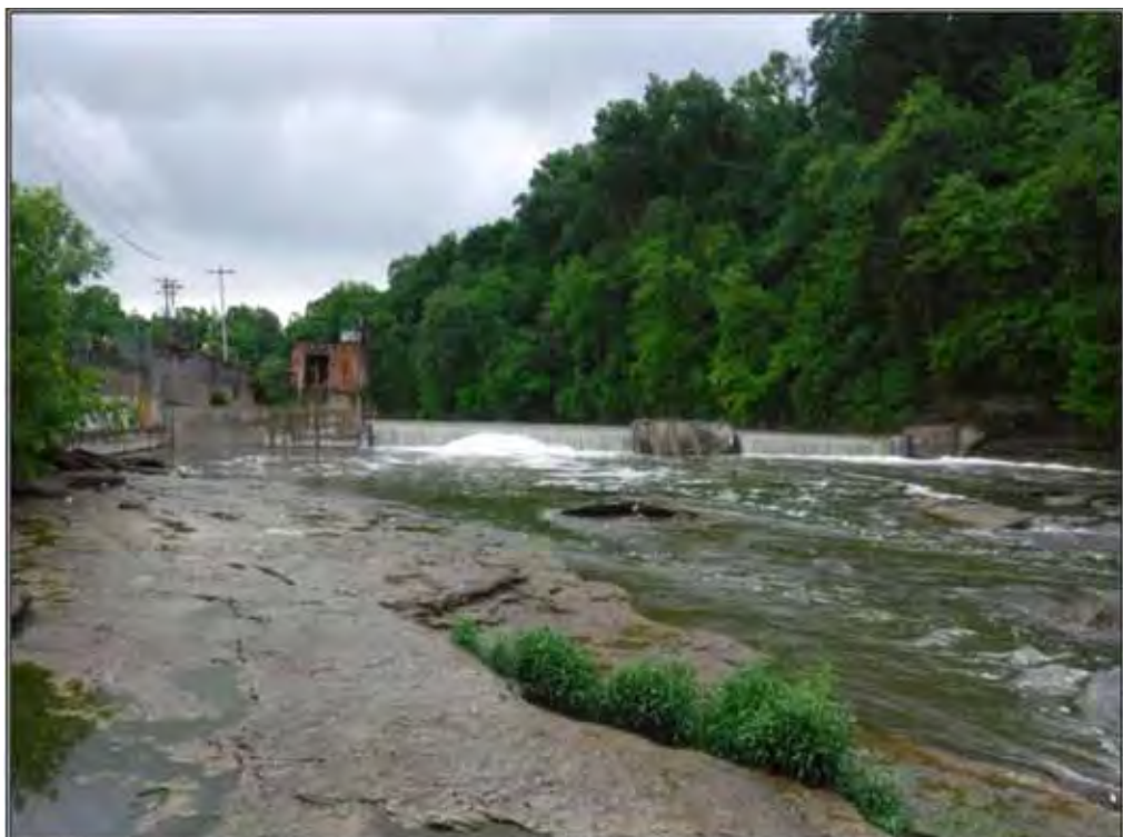
Photograph 1: View of Elkhorn Creek facing upstream towards the low-head dam and pump house. June 23, 2020.
