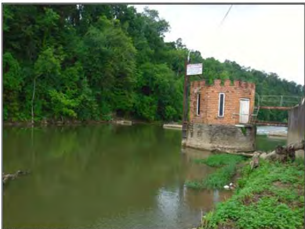
Photograph 2: View of Elkhorn Creek facing downstream towards the low-head dam and pump house. June 23, 2020.
