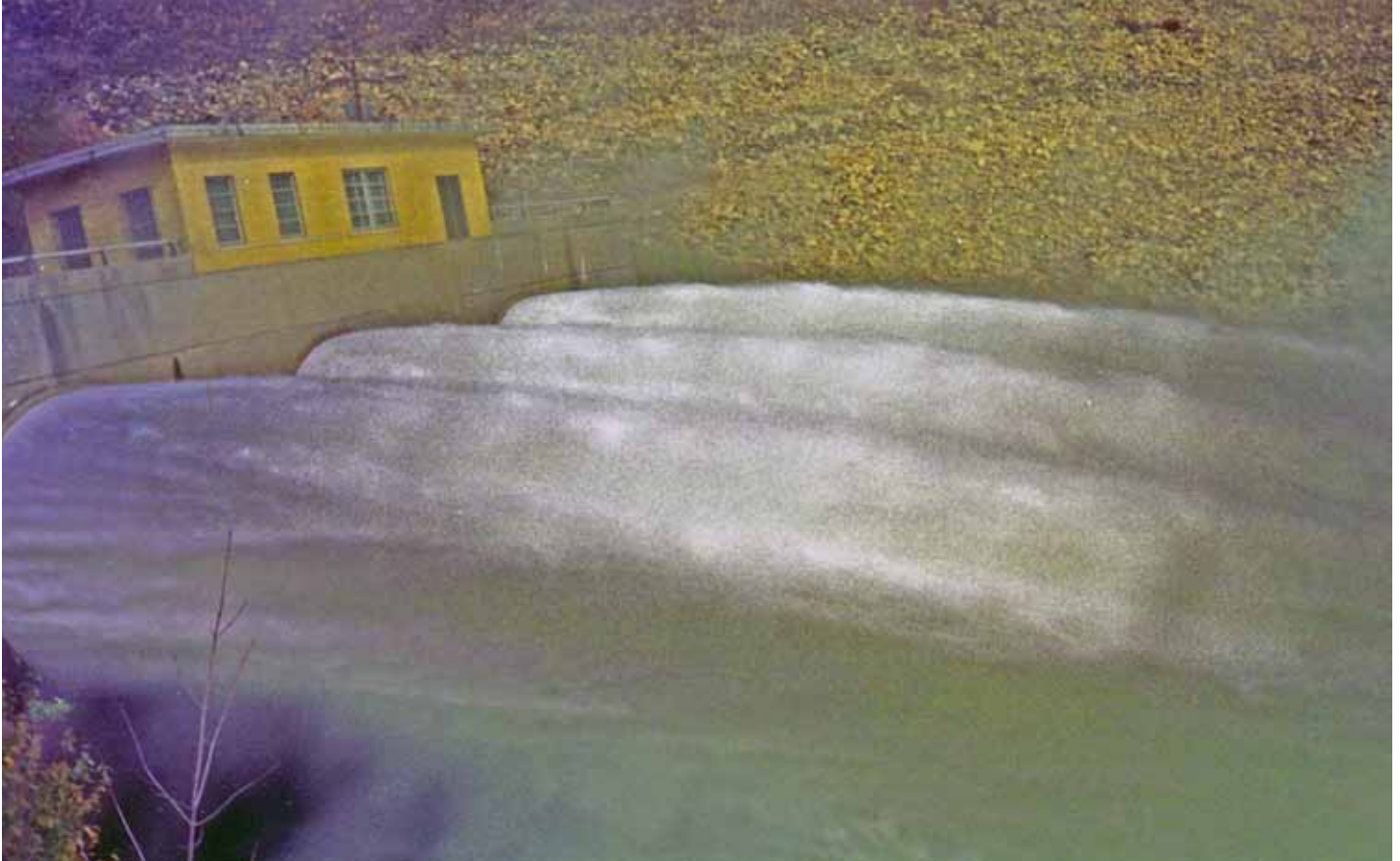
Gauley Dam tubes away!
