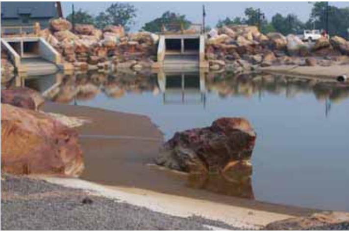
The entry pond showing the pump discharge chutes with the restaurant in the left background.
